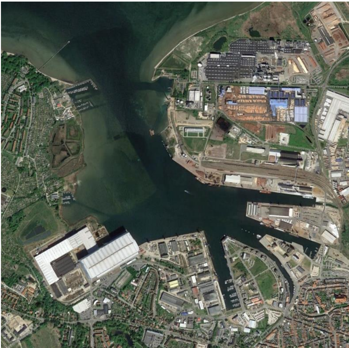
Figure 15 Aerial view of the Port of Wismar.
